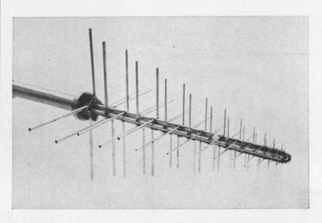
Take two log-periodic antennas, mount them at right angles to each other on a common axis so that their radiation patterns are independent, and the result is an unusually versatile antenna. It combines the broadband characteristic of log-periodics with an ability to provide any field pattern polarization or combination of polarizations.
