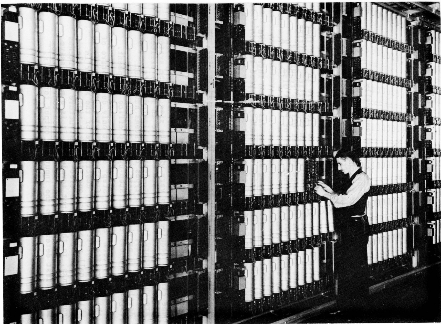
Figure 4-1 Typical Step-by-Step Dial Office Equipment
