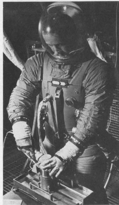
Astronaut uses electron-beam gun to weld stainless steel in chamber that simulates conditions 380,000 feet up.
