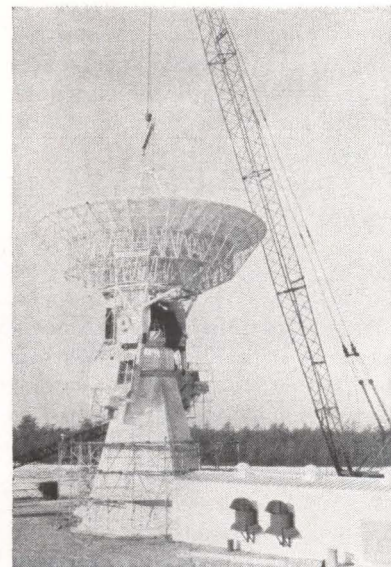
Reflector is lowered onto pedestal
