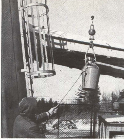
MASER dewar being hoisted to antenna
