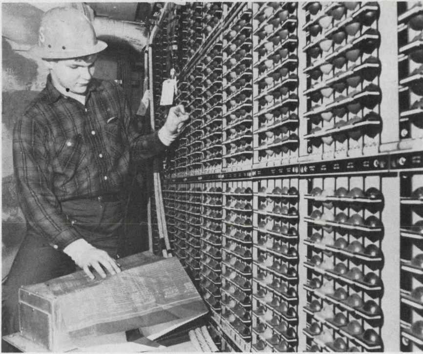
Hunt. Workman checks out Jersey's old receiver patch panel.
